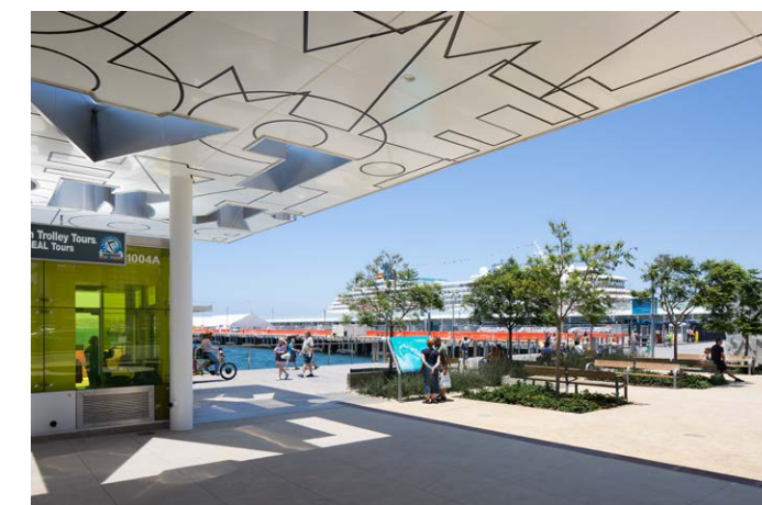
North Embarcadero Pavilion
